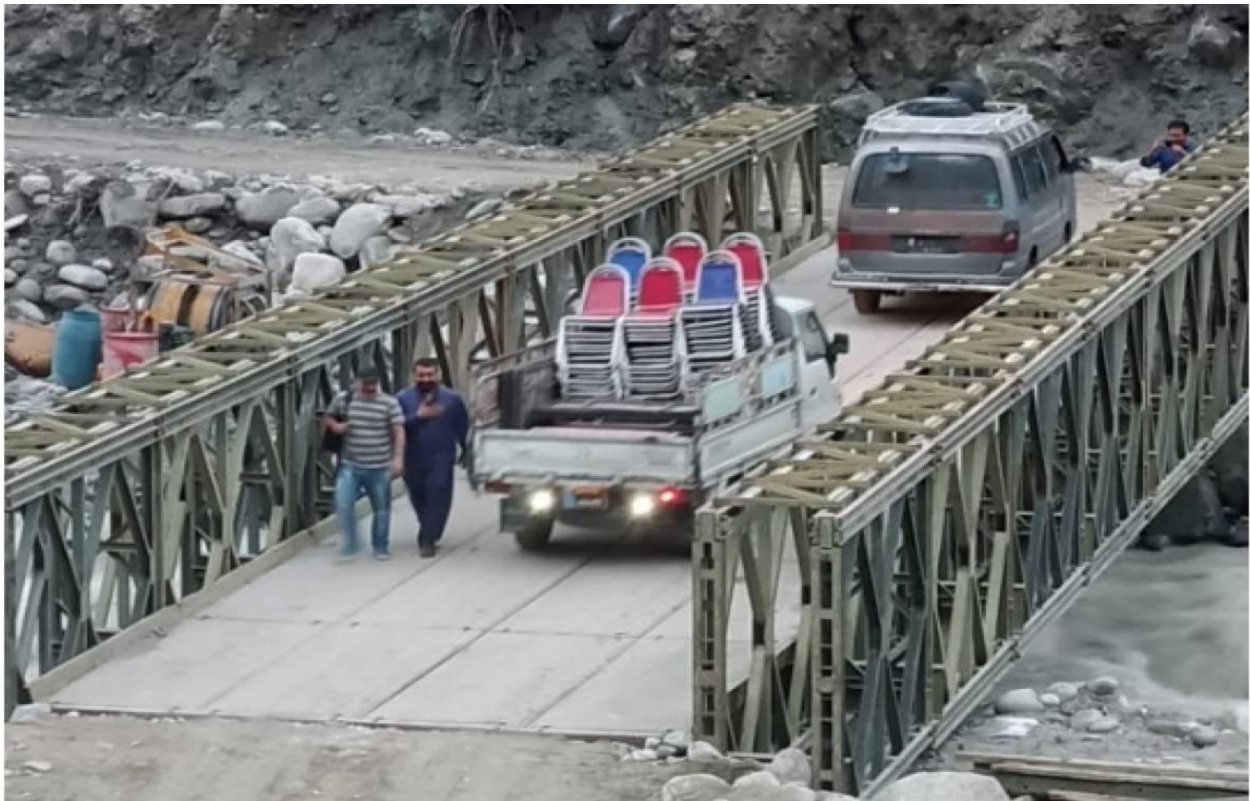
FIGURE 17: RESTORATION OF STEEL BRIDGE (20 MAY 2022)
