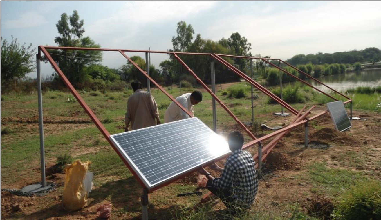
Figure 3.7: Each PV Modules 200 Watts.
