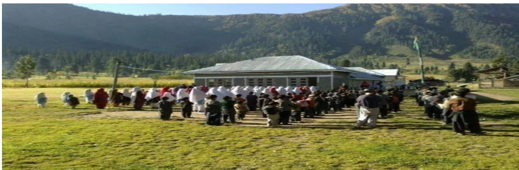
Fig 4.1 Primary school made up of stone structure at arrang kel
