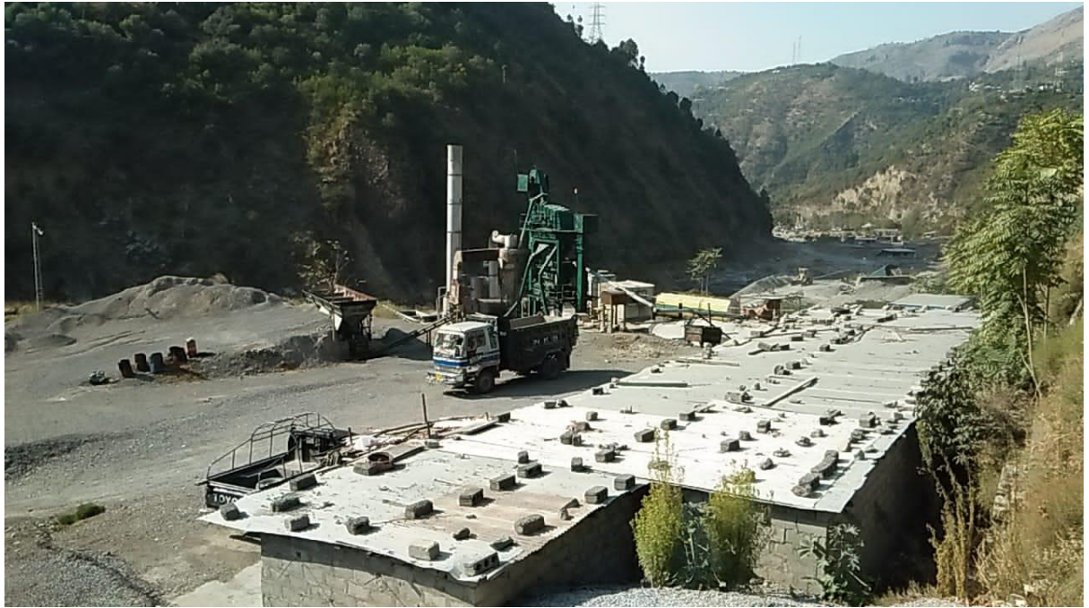
Figure: 5.10 unplanned Infrastructure
