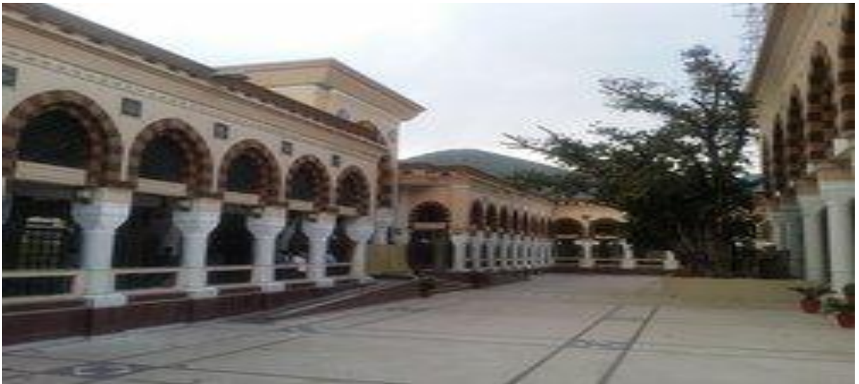
Figure 1;Insider view of new constructed shrine
