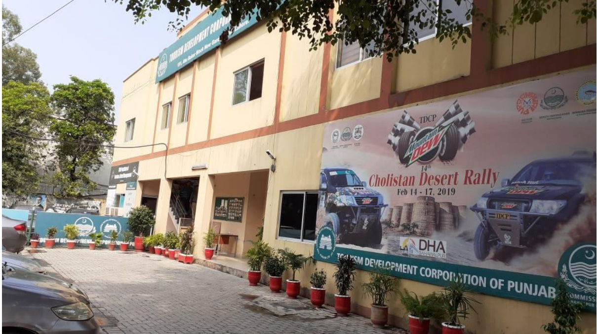
Locale Picture 1: TDCP Head Office, Garden Town Lahore
