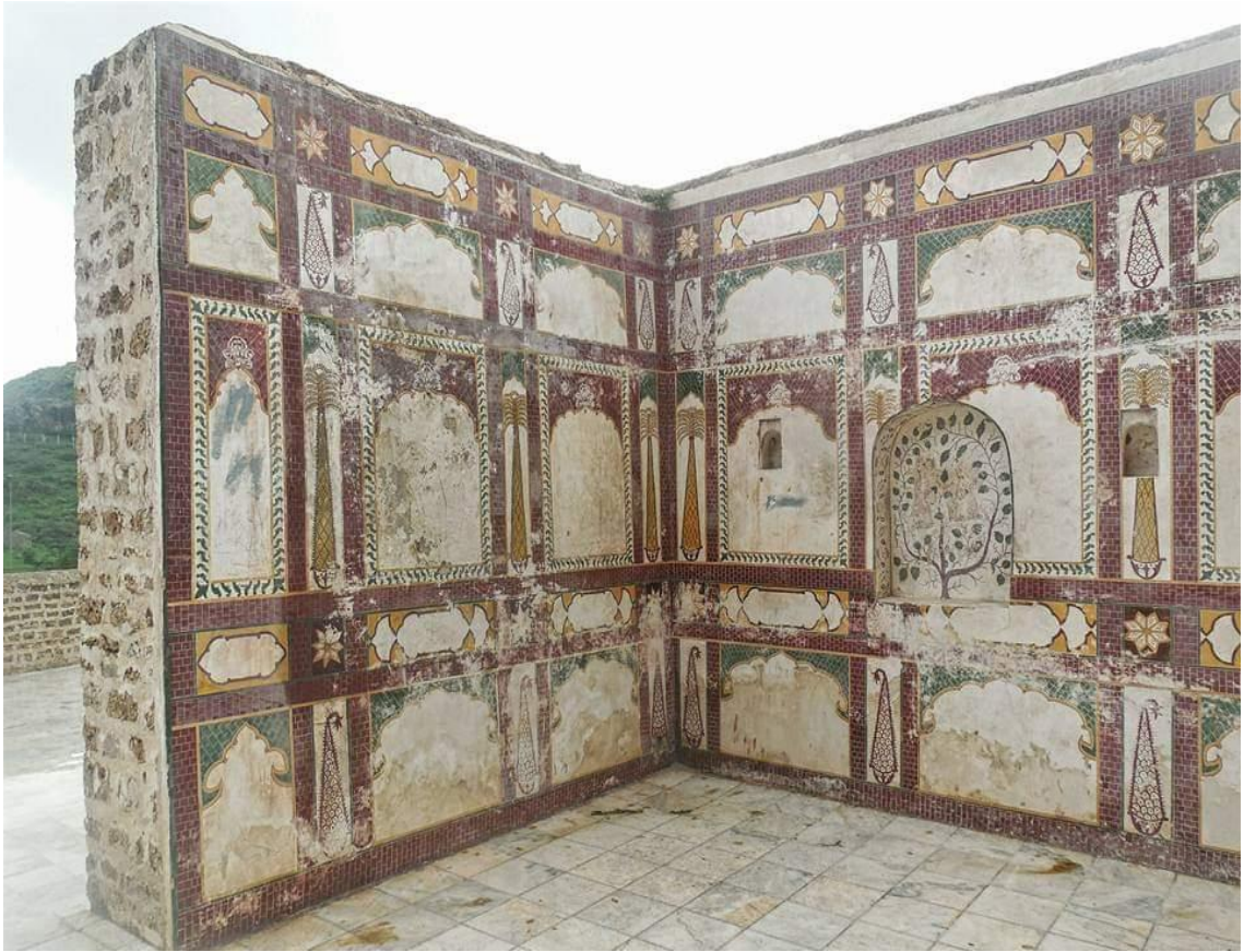
Picture 3: A view of semi-restored walls at the Hari Singh haveli
