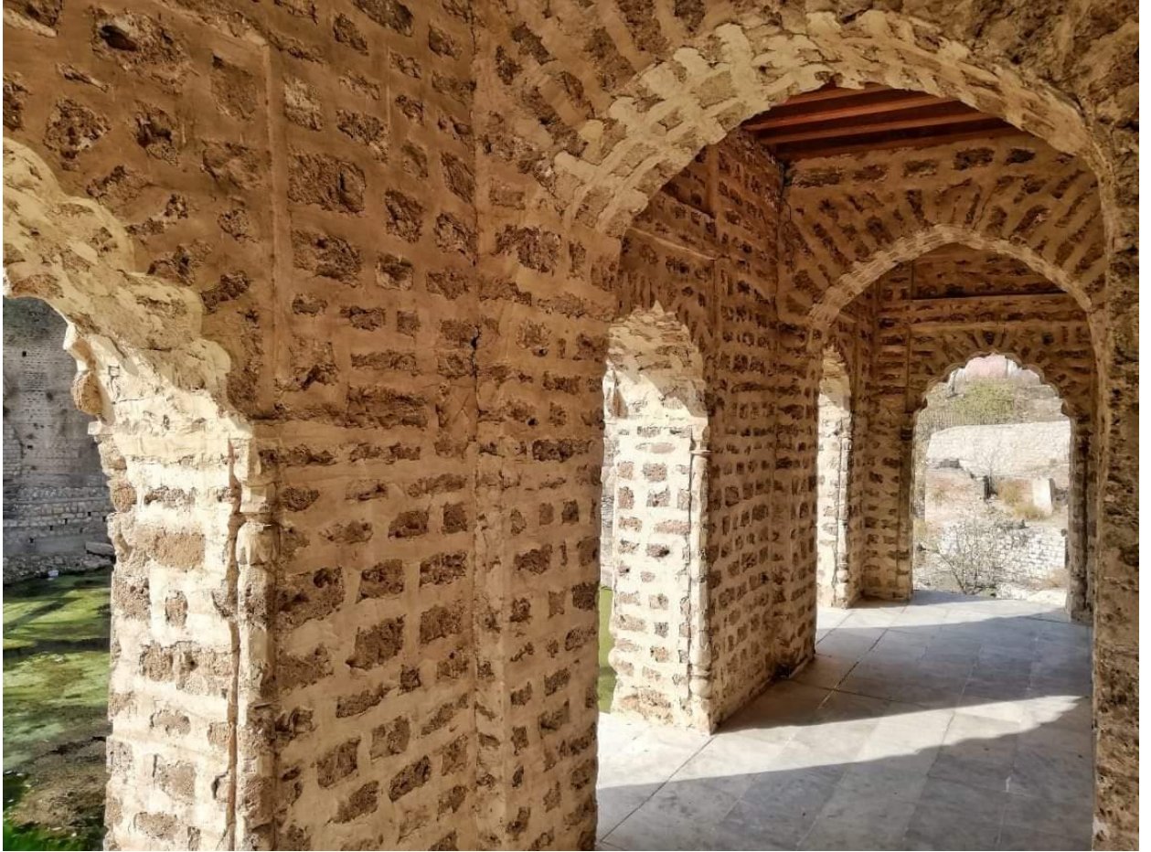
Picture 15: Arched Entrance
